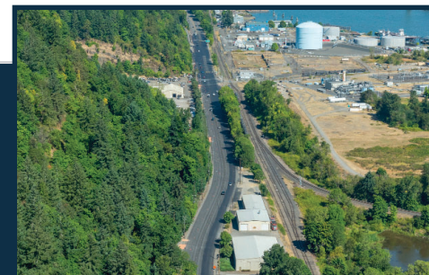
An aerial shot of U.S. 30 during construction.
