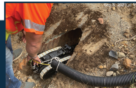
Crews guide camera into culvert to assess conditions.
